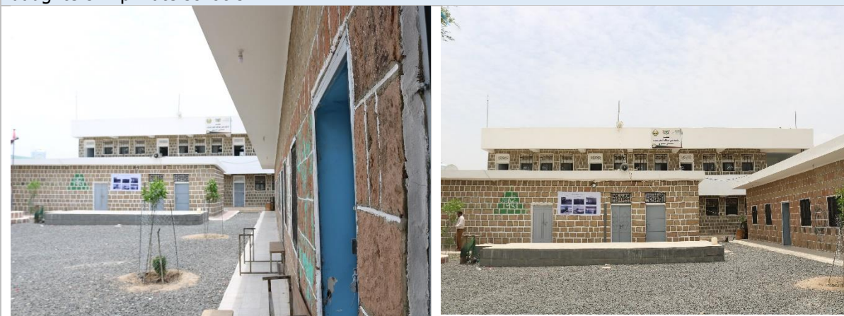
The conditions of Al-Shaheed Albahr school for girls after rehabilitation works. Photo credit: UNDP Yemen/2022.
