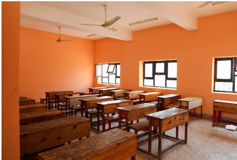
A classroom in Idrees Hanbala school after the rehabilitation works. | Photo credit: UNDP Yemen / 2022
