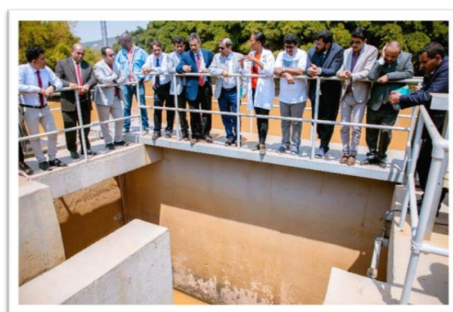
The participants of Exchange Visit visited water treatment plant on 26 August 2022. Photo credit: Resonate! Yemen/2022.
